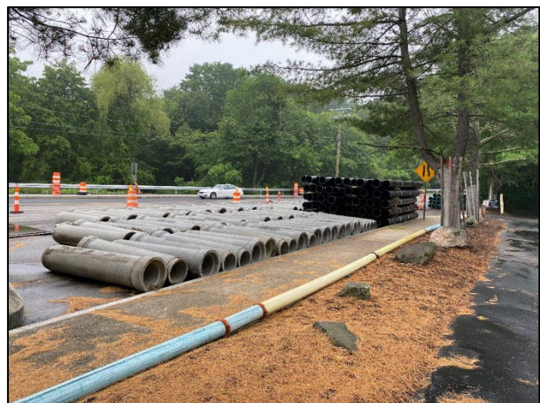
Storage of Pipe Materials with Temporary Water Bypass Piping
