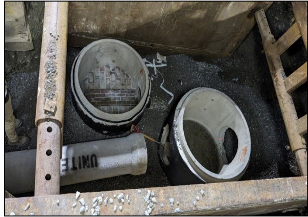
Replacement of Municipal Sewer and Drain Lines on Lexington Street
