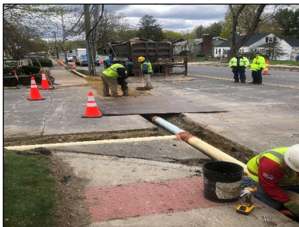
Installing Temporary Water Bypass Piping on Lexington Street
